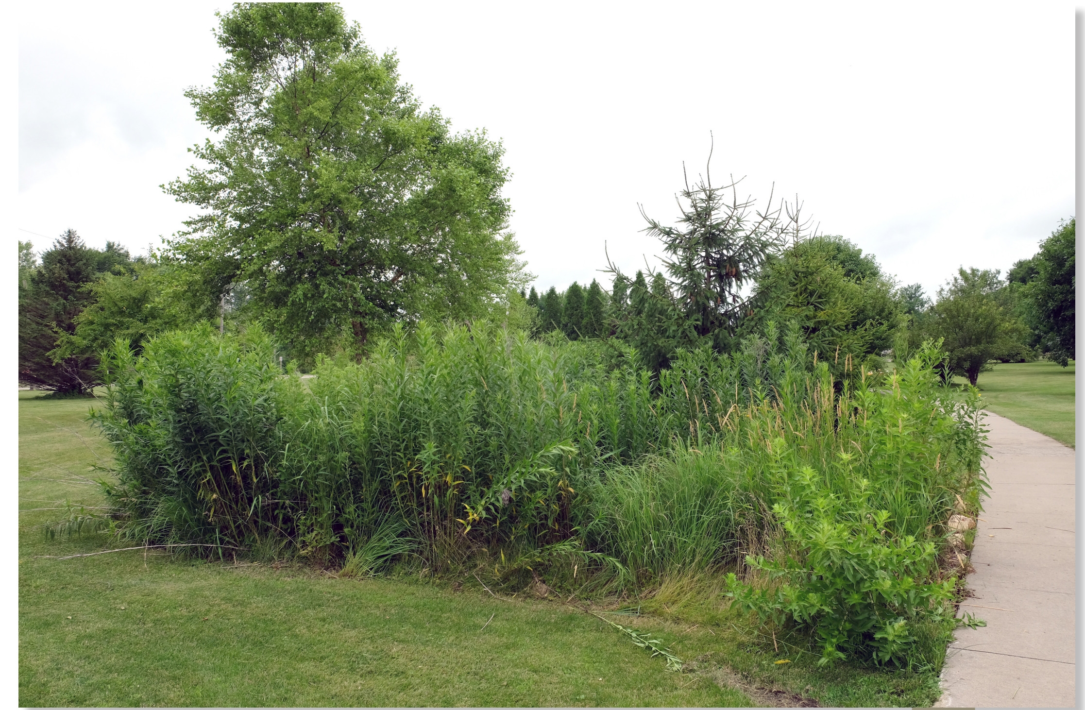
Completed bioswale and new sidewalk, 2016
